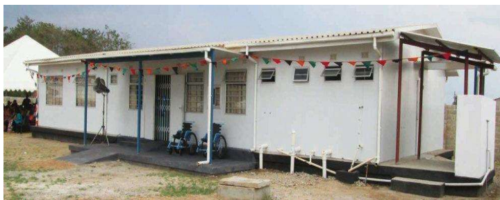
Figure 12 New Maternity Ward at Mahatma Gandhi Memorial Clinic, Kabwe
