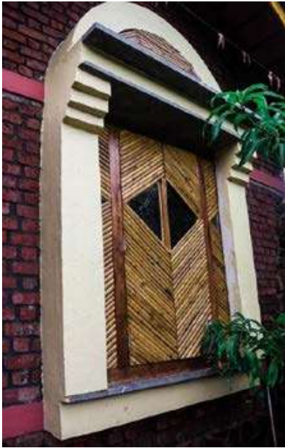
Image 10 – The waste wood window with split bamboo.
