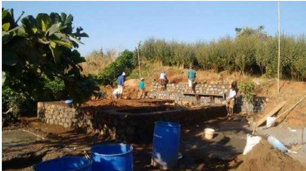
Image 06 – The pre-construction slope after growing tur and vetiver grass on the top level.
