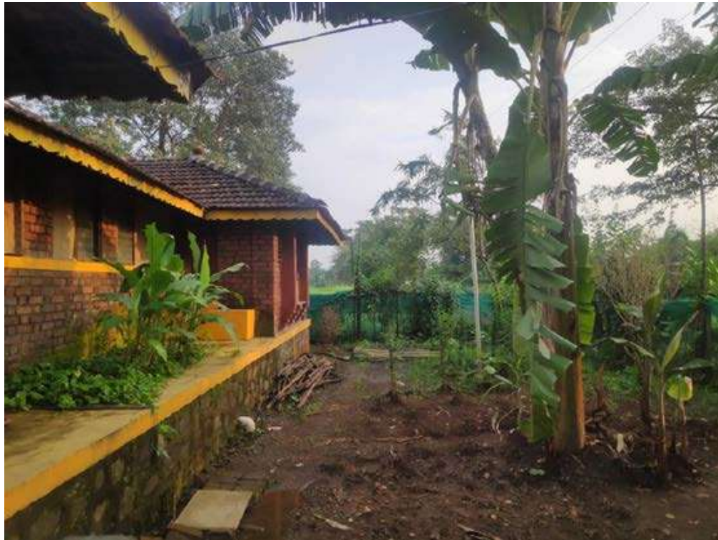
Image 03 – Backyard garden and waste water system.
