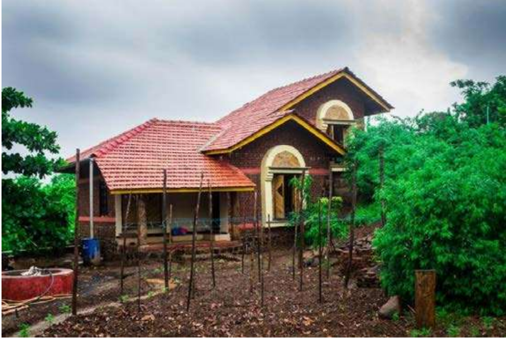
Image 09 – Rain water harvesting and borewell recharge.
